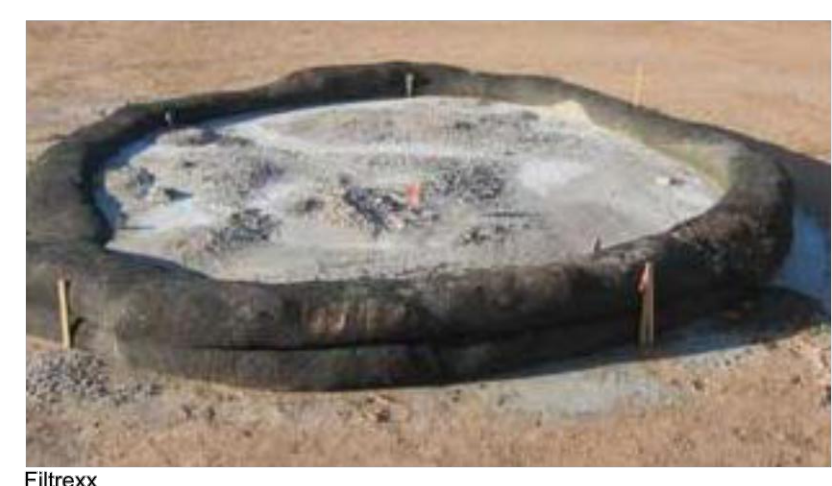
FIGURE 3.18 Typical Composite Sock Washout Installation
